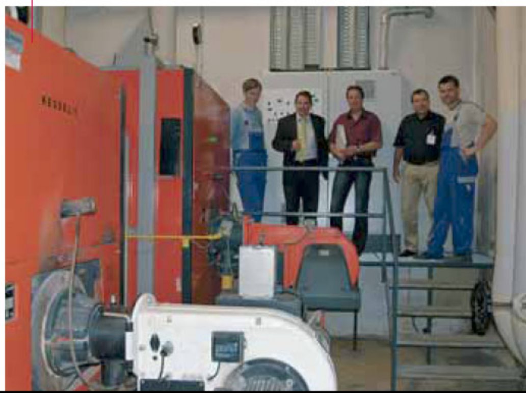
In der alten Heizzentrale. In the old heat station.
